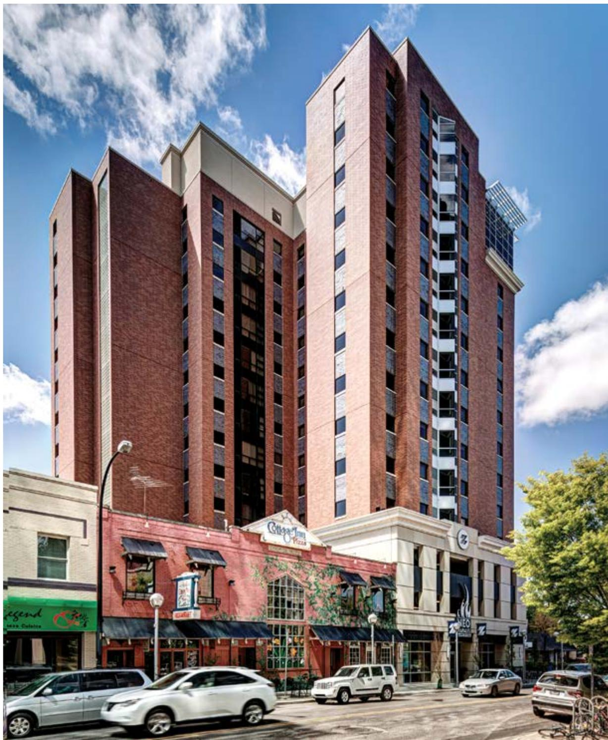
neighborhood and create an iconic appearance. The exterior shell features cast-in-place concrete on the lower three levels of retail and parking with load-bearing precast concrete walls and floors above.
